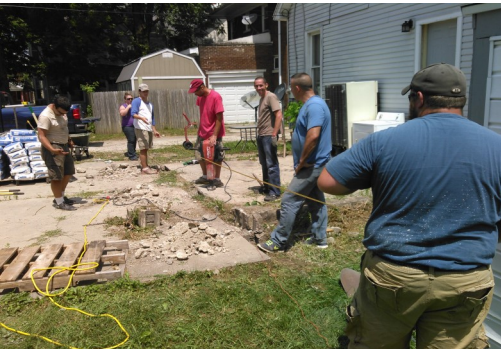
Digging post holes for privacy fence
