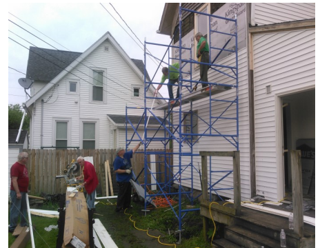
Ohio mission team putting on siding.
