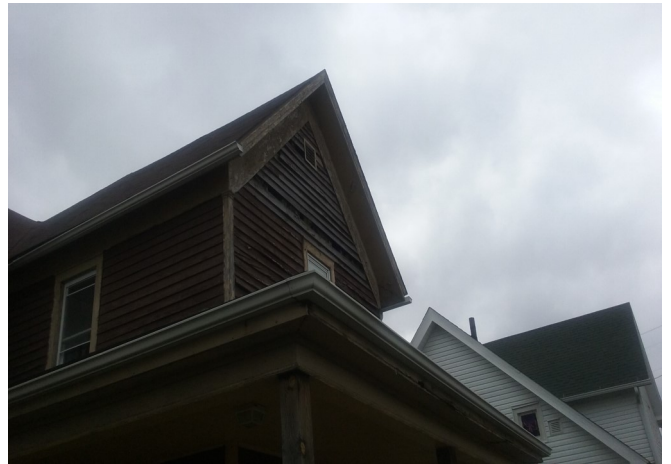
Repairs and vinyl siding .
