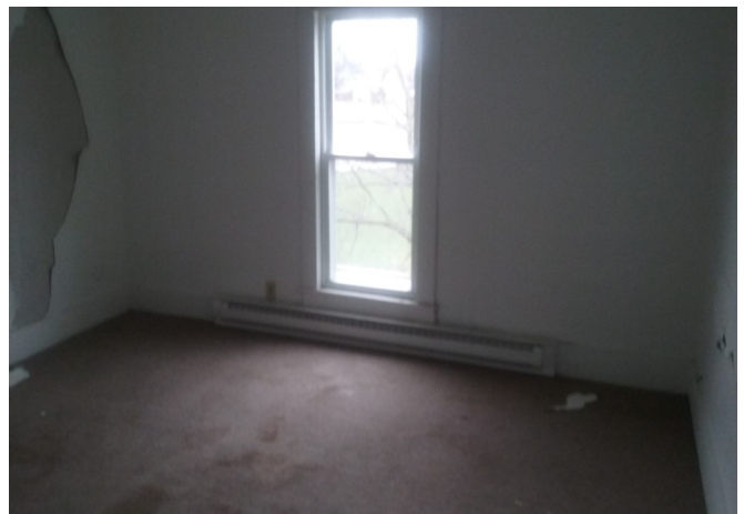
Take out carpet throughout house and restore floors.
